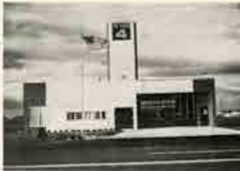
fig. 10 Venturi and Rauch, Fire Station No. 4, Columbus, Indiana, 1965.
