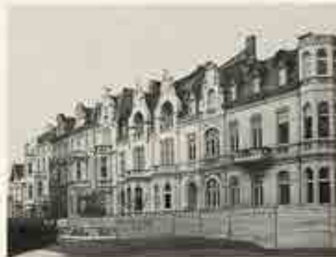
← fig. 2 Bonn, Südstadt district. Simrock-Strasse before its demolition. A bank headquarters swallows one hundred apartments. (Photo: Waldemar Haberey, Bonn)
