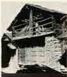
Fig. 6 Attic in Bruson (Valais, Switzerland).
