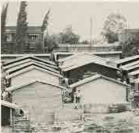
figs. 5–6 “Company houses,” that is, cooperative housing, Nairobi.
