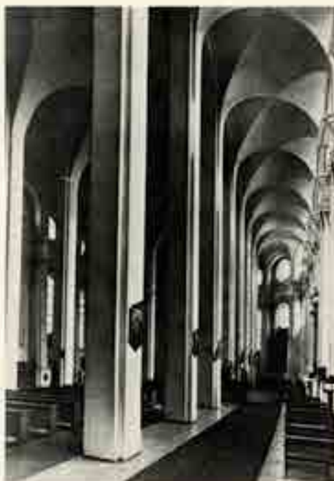
Fig. 7 Munich, Heiliggeistkirche after its "restoration" of 1952.
