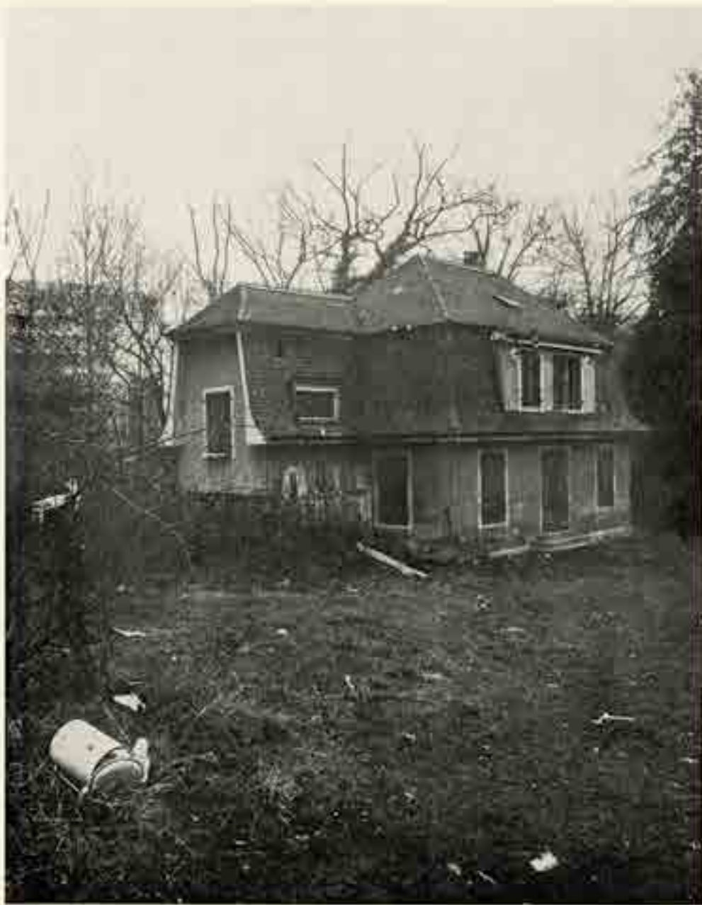
↓ fig. 1 Abandoned villa inhabited by seasonal and annual workers in the Grottes district, Geneva.
