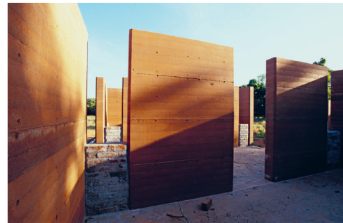
FIG. 3 Earth construction is a common example of an age-old residential construction technology that is, unfortunately, no longer permissible under most building codes. Yet, the method is inexpensive and more than adequate (structurally and climatically) - especially when you consider the unmet needs of hundreds of millions of people. Photo: Andreas Delfino
