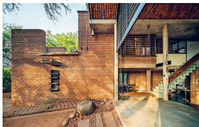
FIG. 2 Wall House (Auzoville, 1996) was a living laboratory that housed a decade of building technology experiments and prototyping. From 1" thick, pre-industrial schikal bricks, to vaulted brick and terracotta roofs, to coffered/filler concrete slabs, to innovative spaces and volumes, the Wall House has explored a range of building technologies using common materials and products (not typically used in building construction) in unexpected ways. The laboratory helped train a community of craftsmen who have since gone on to build commercially thriving construction ventures. Photo: Javier Callejas
