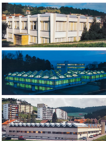
The Caractères SA factory at Rue du Parc, Le Locle, in an advertising brochure from Caractères SA for injection-moulding tools and parts, 1987. Unknown photographer
